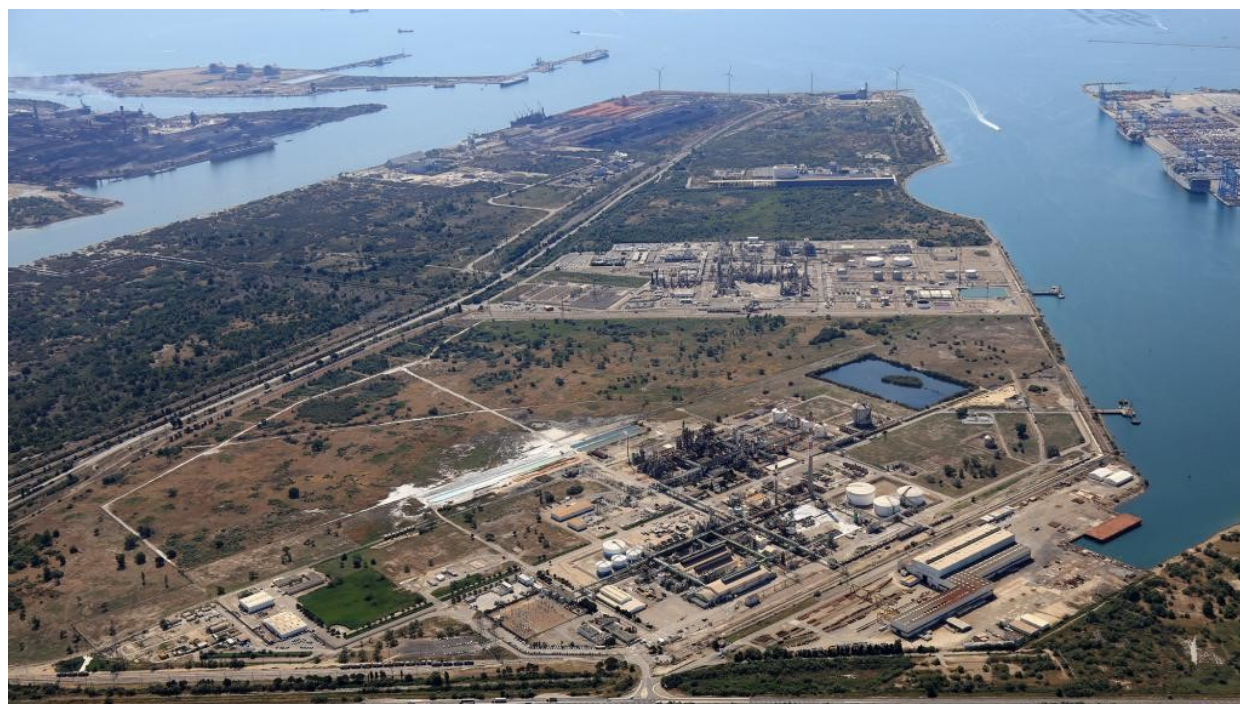
The port at Marseille
